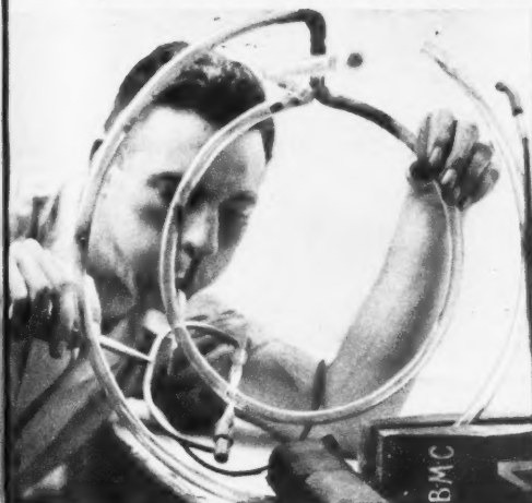
To splice two ends of glass tubing together into a perfect circle, the blower uses a special torch. Below, craftsman puts the electrode in the tube.
